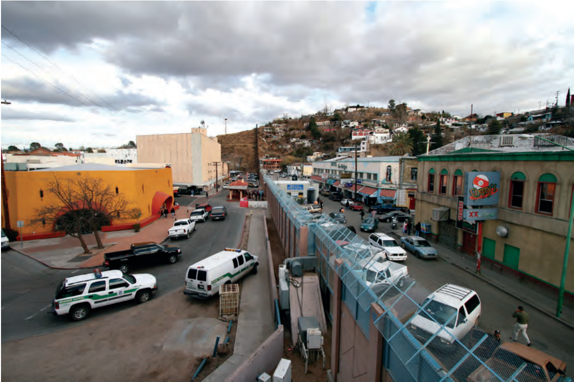
In 2007 the towns of Nogales, Arizona (United States), left, and Nogales, Sonora (Mexico), stand separated by a concrete and steel fence. (U.S. Army/ Gordon Hyde)
