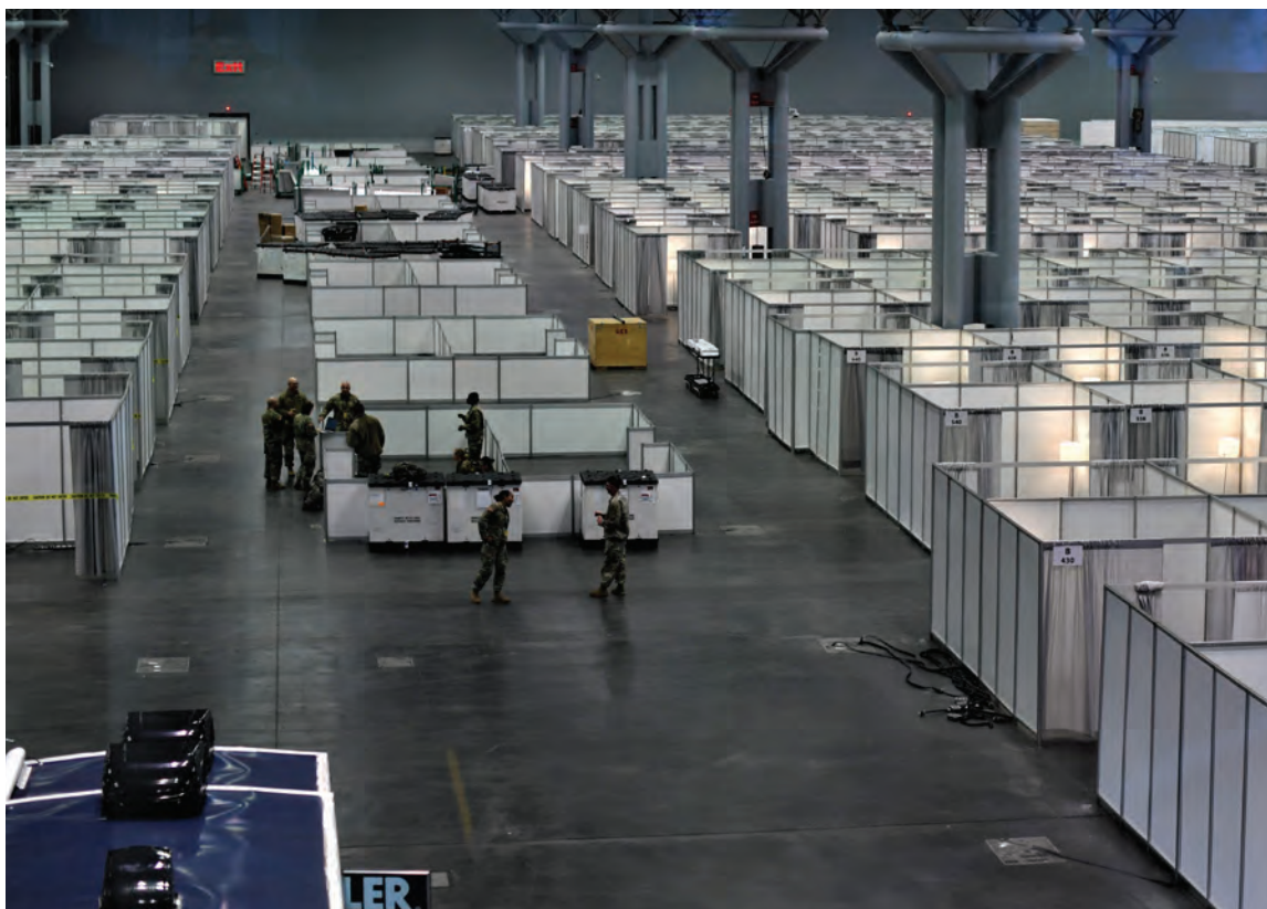
Military members begin adding lamps to the Patient Care Units (PCU) for Phase II at the Jacob K. Javits Convention Center in New York City. (Photo by New York National Guard, April 2, 2020)
