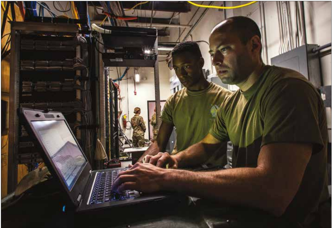
South Carolina Army National Guardsmen from 228 th Signal Brigade out of Spartanburg, South Carolina, set up Joint Incident Site Command Center package to support Horry County Emergency Operations Center with back-up communications system, September 15, 2018 (U.S. Army National Guard/ Brian Calhoun)
