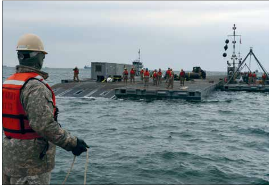
Soldier assigned to 331 st Transportation Company works to bring last sections of Trident causeway together during Combined Joint Logistics Over-the-Shore military exercise on the Korean Peninsula, April 18–28, 2013 (U.S. Navy/Anthony R. Hayes)
