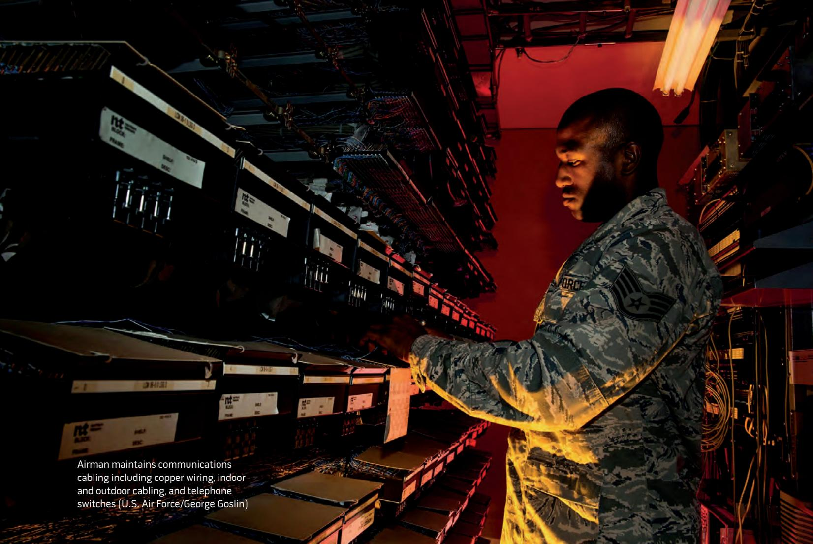
Airman maintains communications cabling including copper wiring, indoor and outdoor cabling, and telephone switches (U.S. Air Force/George Goslin)
