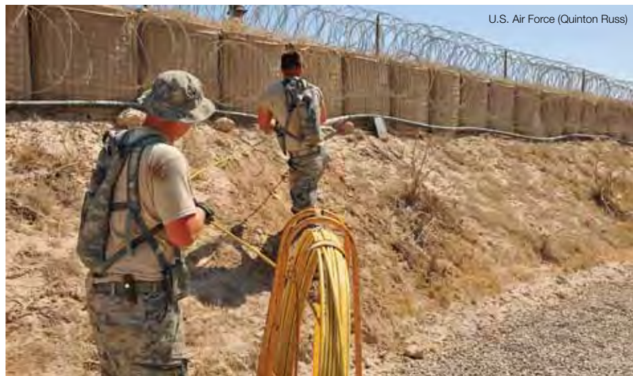
Airmen prepare to run fiber optic cables to improve connectivity at Camp Herat, Afghanistan
