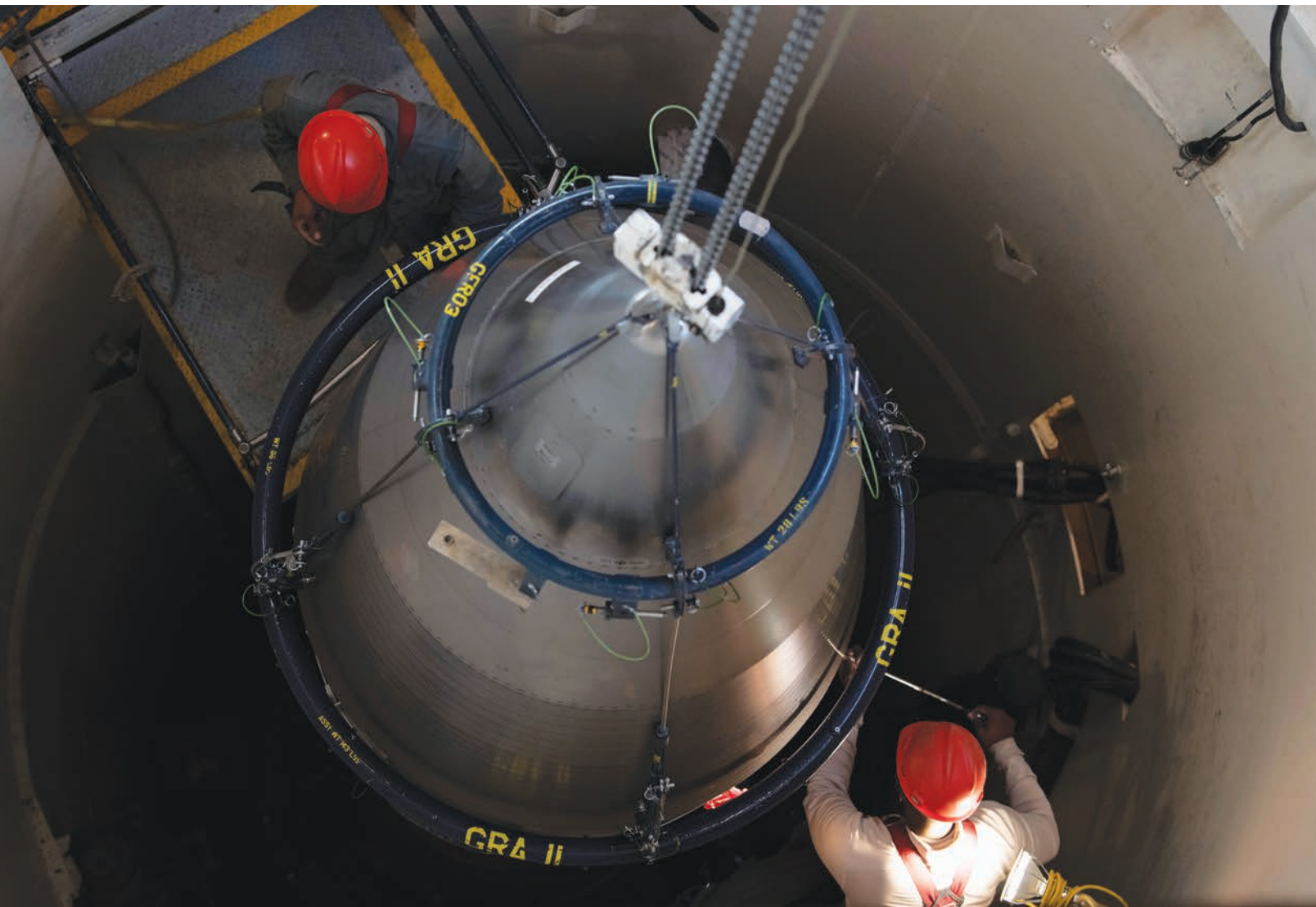
Airmen from 90 th Maintenance Group maintain and repair intercontinental ballistic missiles on alert status, December 18, 2019, within Francis E. Warren Air Force Base, as part of Air Force Global Strike Command (U.S. Air Force/Abbigayle Williams)
