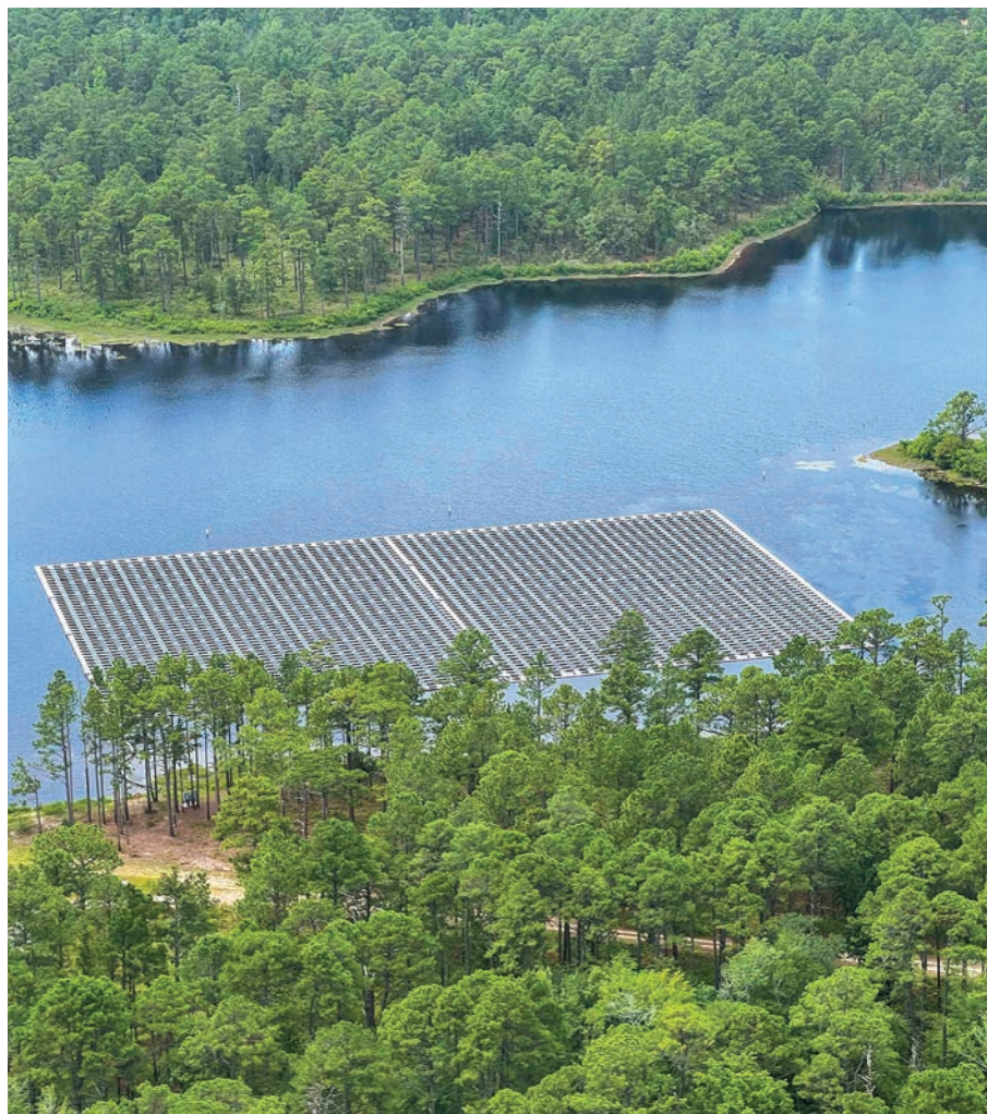
Floating solar microgrid consisting of 2,700 solar panels on lake at nearby Camp Mackall provides clean energy to Fort Liberty, North Carolina, July 28, 2023 (U.S. Army/Jason Ragucci)
