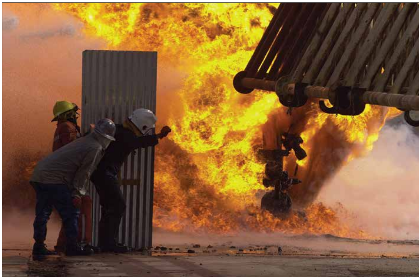
Kuwaiti oil well control specialists direct fire control rig over oil well fire in order to complete water blasting method to extinguish fire at Rumaila Oil Field, in southern Iraq, as part of Operation Iraqi Freedom , March 27, 2003 (U.S. Army/James P. Johnson)
