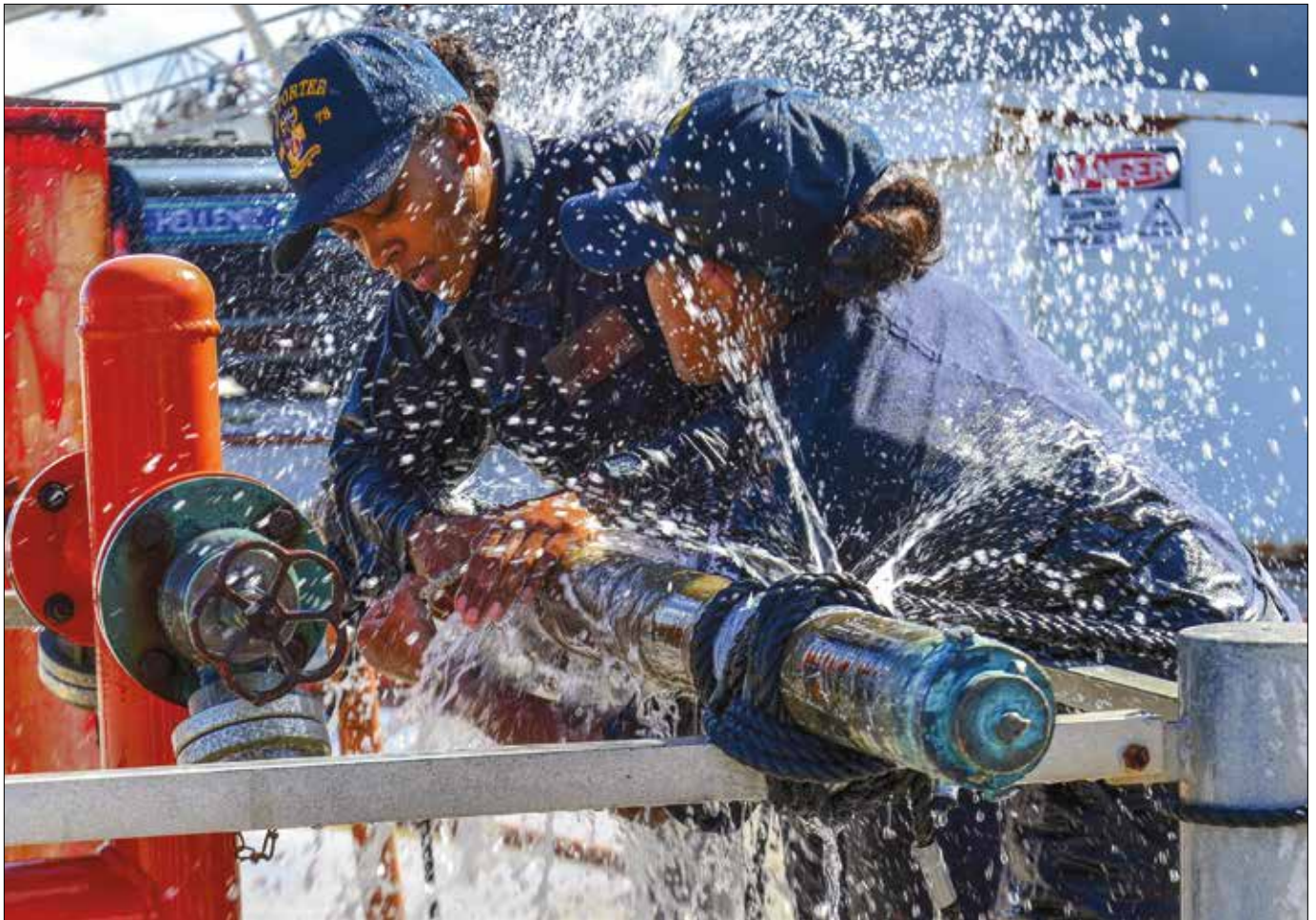
Sailors assigned to USS Porter apply jubilee pipe patch during damage control competition at Naval Support Activity Souda Bay, Greece, October 24, 2017 (U.S. Navy/Krystina Coffey)
