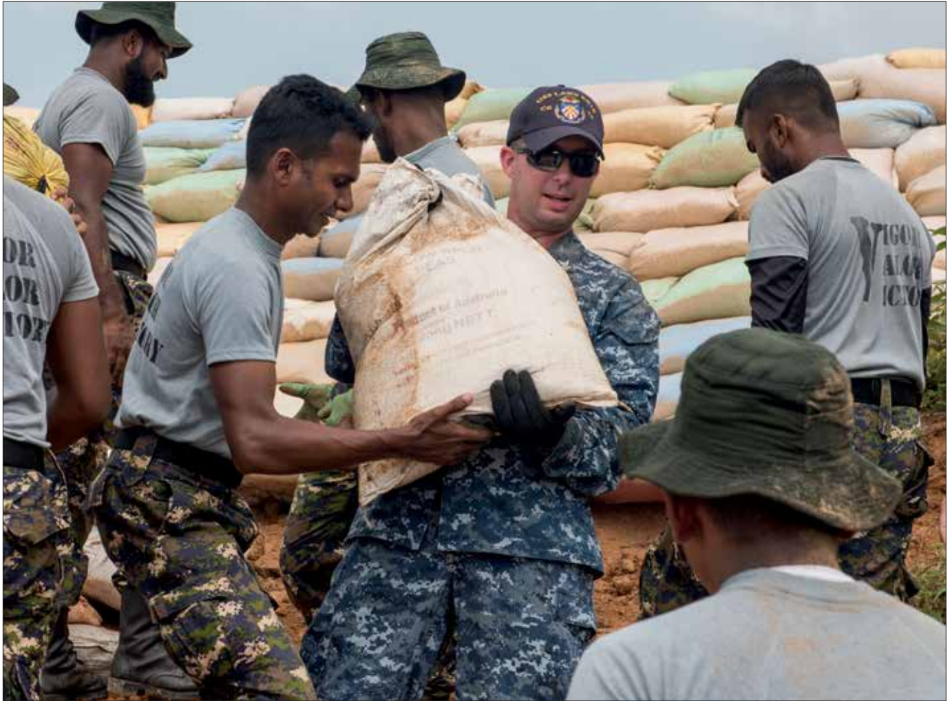
Fire Controlman from USS Lake Erie works with Sri Lankan marines to repair levees in Matara, Sri Lanka, during humanitarian assistance operations in wake of severe flooding and landslides, June 12, 2017 (U.S. Navy/Joshua Fulton)
