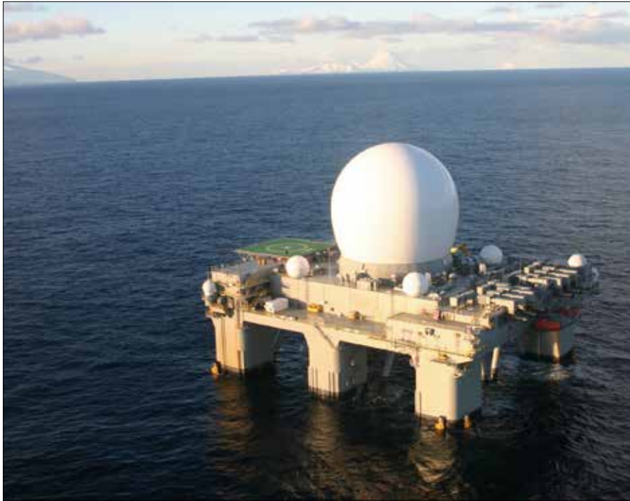
Sea-Based X-Band radar successfully traveled from Pearl Harbor, Hawaii, to waters off Aleutian Island chain of Alaska, February 2007 (Missile Defense Agency)
