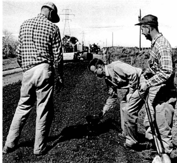
Figure 4. The Author Helping Build a Test Road in Central Missouri Using His Technical Findings From the Lab
