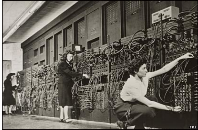
Figure 2. Programming the ENIAC by moving connecting cables by hand
